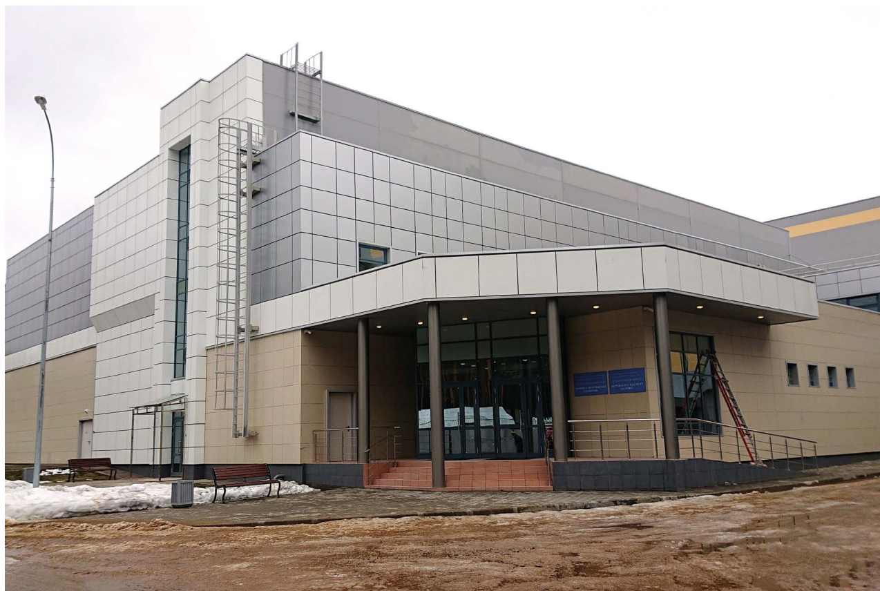
Fig. 5. The building of the experimental complex "Factory of superheavy elements" (SHE-factory).
