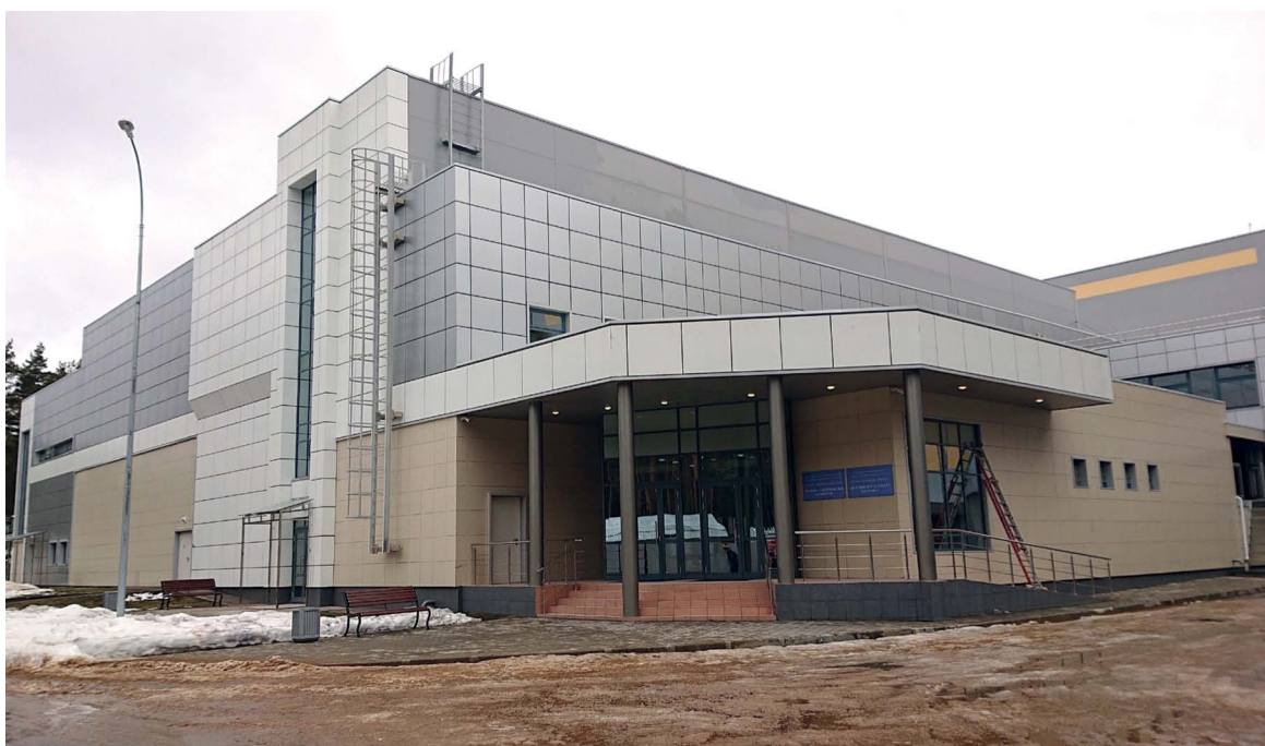
Fig. 5. The building of the experimental complex “Factory of superheavy elements” (SHE-factory).
